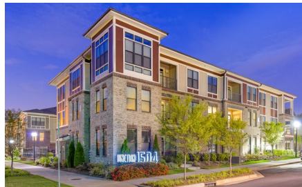
Junction 1504 Apartments Residential | Charlotte, NC
